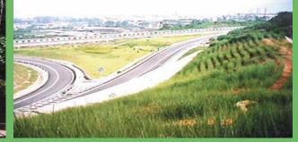
China - expressway stabilization. This cut was prone to massive slip. Stabilization with VS has given complete protection
