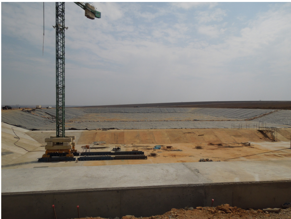
Figure 4-4: Construction progress on the Station Dirty Dam as of 11 September 2013
