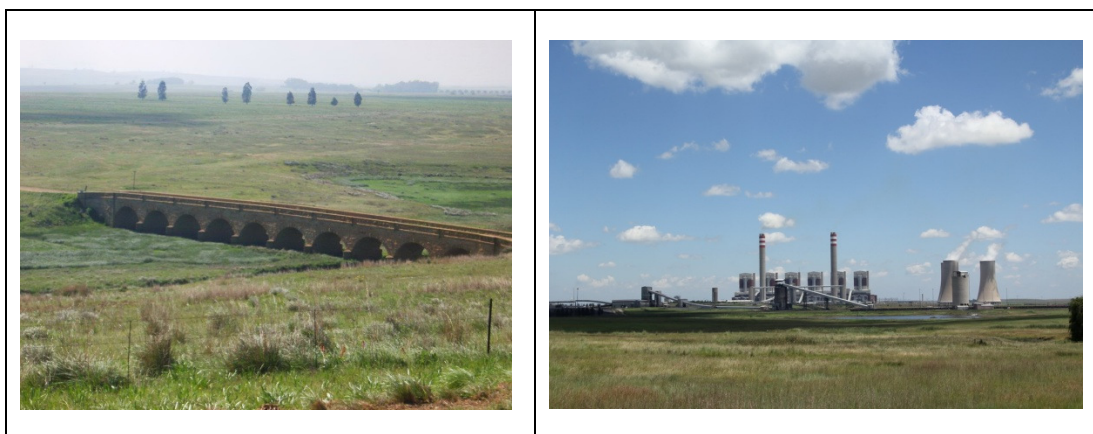
Fig. 7. An old bridge across the Vaal River and Majuba Power Station.
