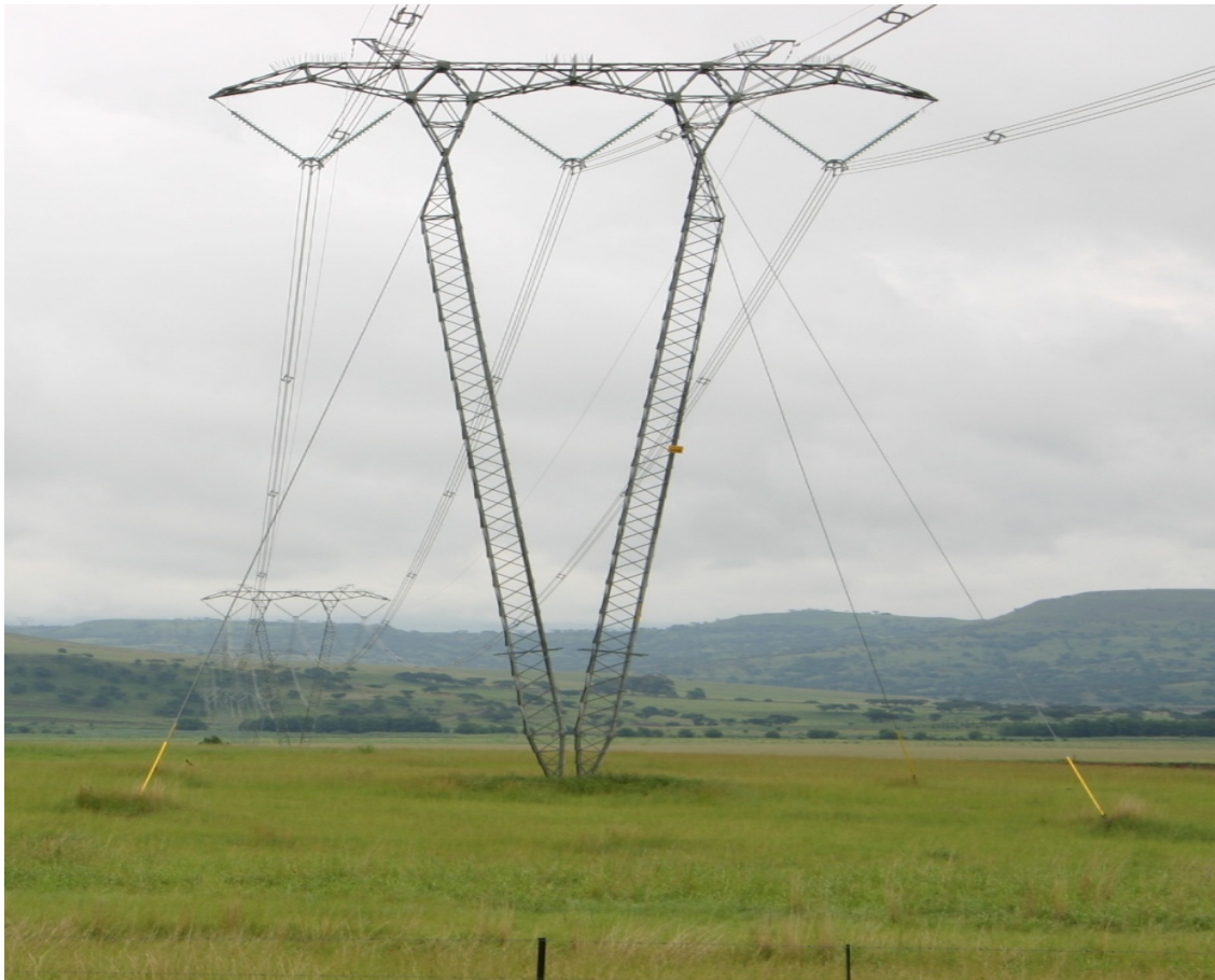
Figure 10: Guyed V 400kV Tower Design
