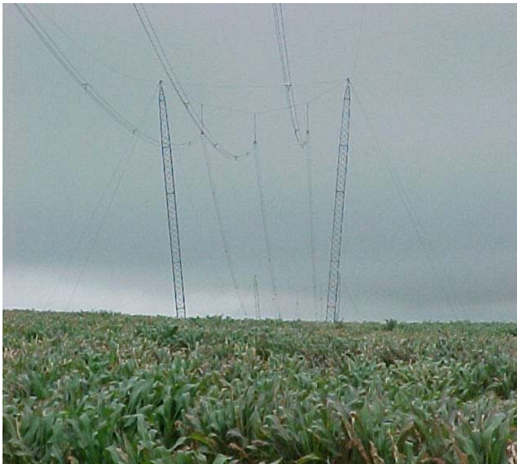
Figure 12: Cross-Rope Suspension Tower Design
