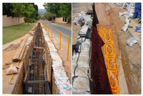
Figure 2.1: Cable Trenching
