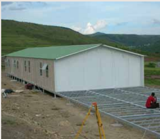
A classroom block under construction.
