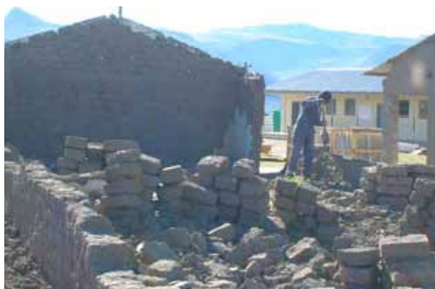
Demolishing some of the unsafe mud structures.
