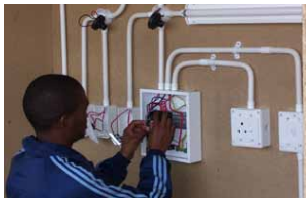
A student doing a practical test on internal wiring.
