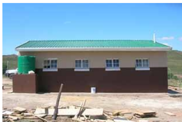
Newly completed ablution block.
