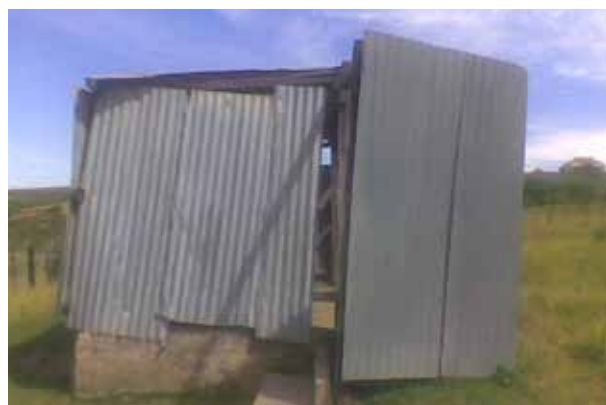
The corrugated iron ablution blocks.
