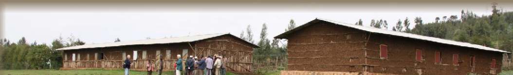
Two additional classrooms constructed with help from the Middelpunt Wetland Trust
