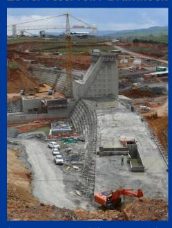
Overall progress is 63% complete. A final lift remains for the intake and outlet tower. Pre-cast gallery roof slabs have been placed and covered with RCC on both right and left bank. 204 027m³ of soft and hard material has been excavated and 18 546m³ concrete has been placed. The placing of RCC is in progress on both flanks with 36 640 m³ placed. The expected date for impoundment is in April 2010 and completion in October 2010.
