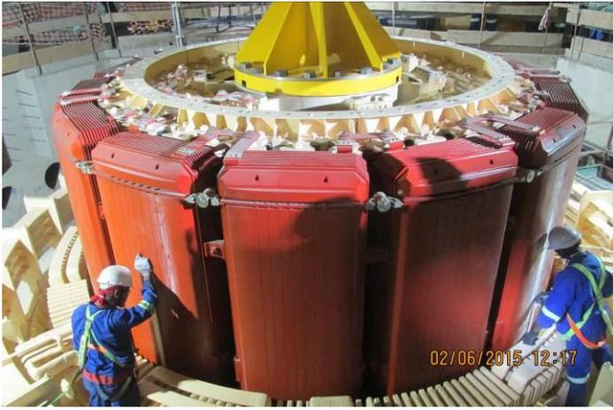
**Rotor being lowered into stator**
