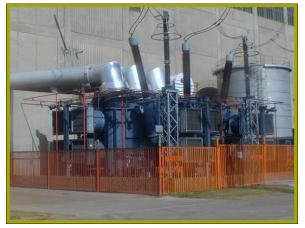
**Photo 10:** Step up transformers. The silver pipes enclose the conduits transporting electricity from the generator to the transformers (painted blue in the photograph)
