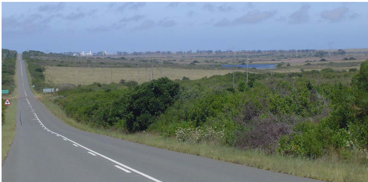
Figure 6.3: Photograph taken travelling south along the R327 towards the Gourikwa power station (seen in the background)
