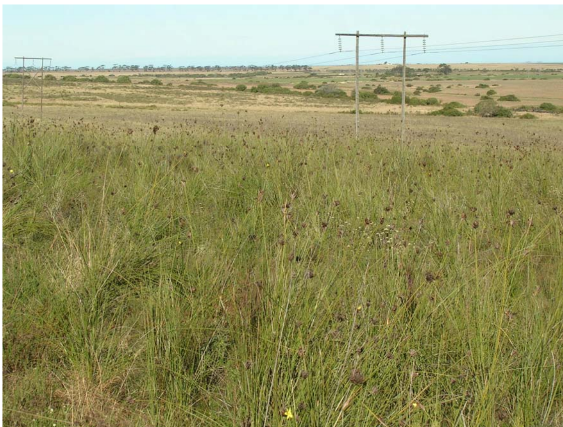
Figure 5.3: View of the area between the Proteus Substation and Gourikwa, crossing mosaic of ploughed lands and Mossel Bay Shale Renosterveld.
