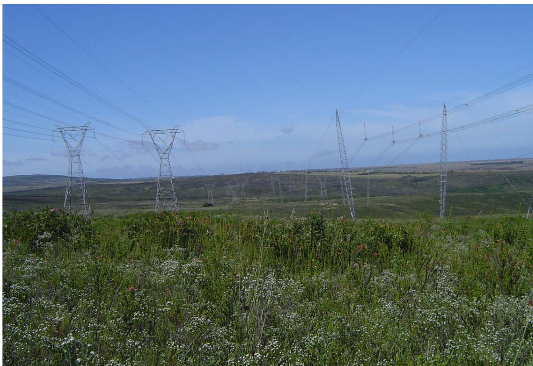
Figure 7.5: View of existing transmission and distribution lines between the Gourikwa Power Station and the Proteus Substation
