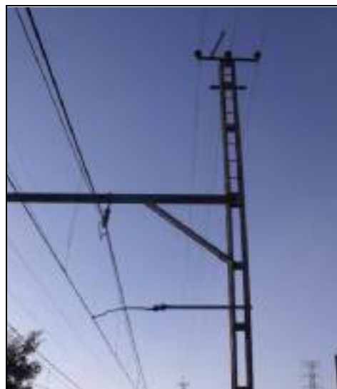
Figure 3-6: Example of the proposed OHTE.
