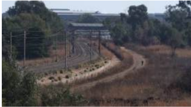
Figure 3-9: Example of an access road.
