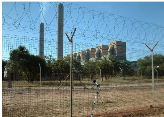
View towards Matimba power station
