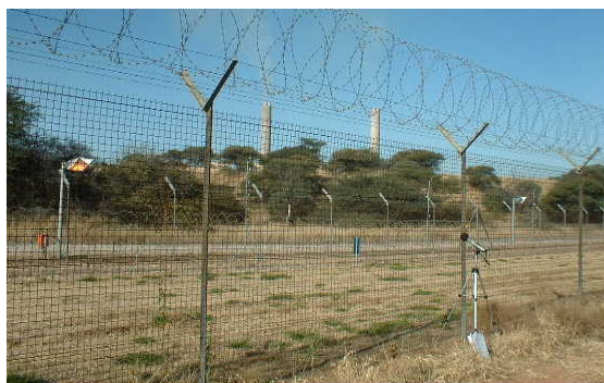
View to Matimba power station which is partly obscured by the existing landfill
