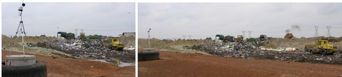
Views towards the reception pit
