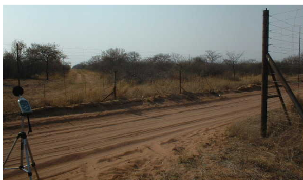
View along fence line between Gannavlake & Loopleegte
