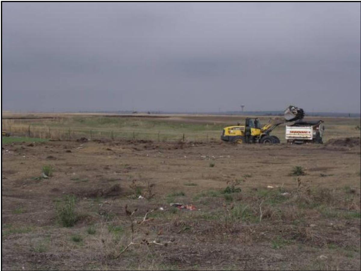
Figure 4-1: Example of what the waste site would look like while operating
