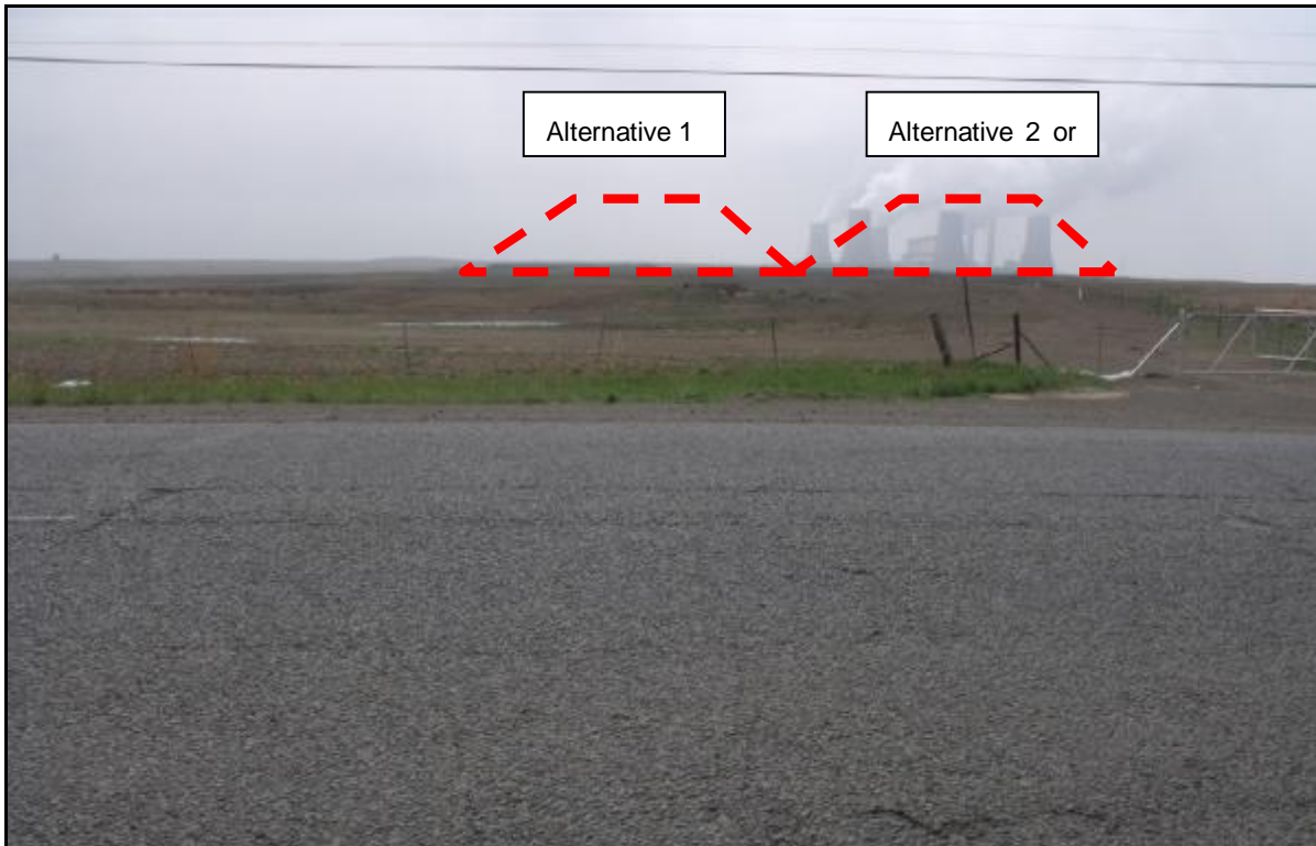
Figure 3-2: View from the New Denmark – Standerton Road illustrating the view of the completed disposal after 40 years.
