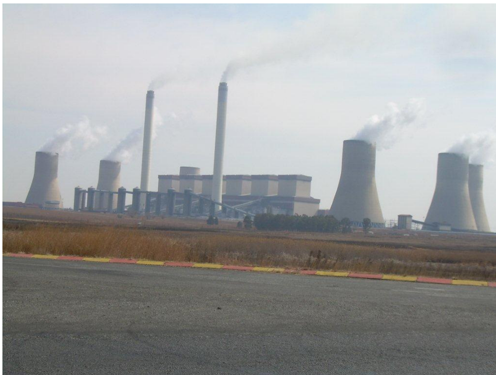
Figure 10.2: Tutuka Power Station forms the centre point of the study area, as the source of ash
