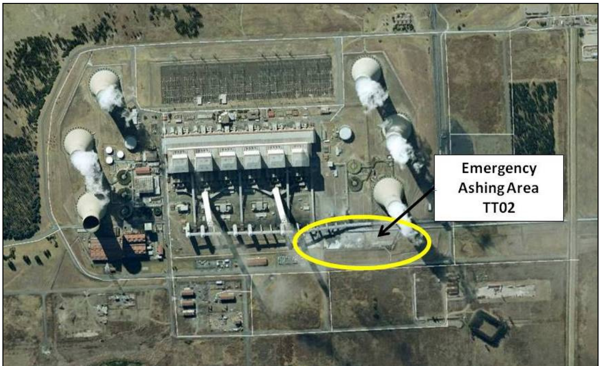
Figure 4.5: The location of the emergency ashing area (TT02) within the Tutuka Power Station Terrace area
