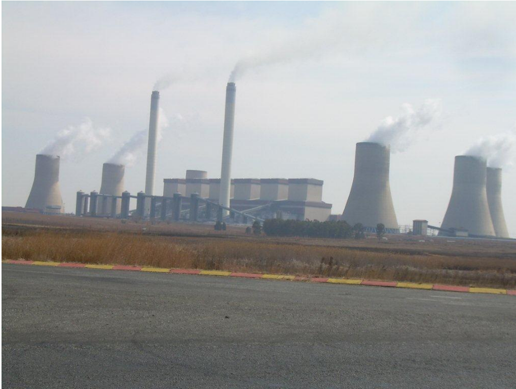
Figure 1: Tutuka Power Station forms the centre point of the study area, as the source of ash
