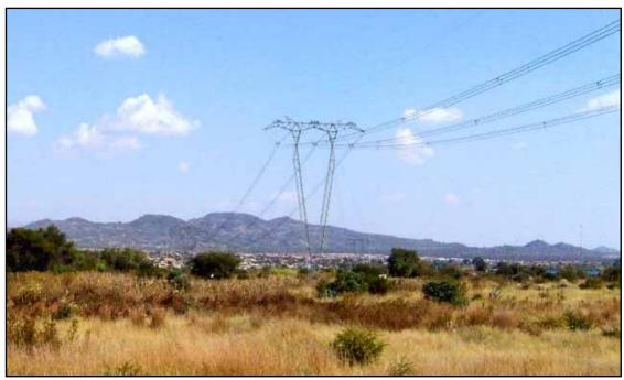
Figure 2.2: Compact Cross-rope suspension tower
