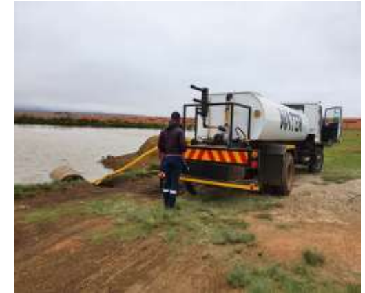
Figure 15: Water abstracted from dam located close to site.
