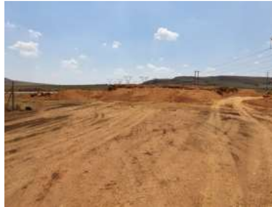
Figure 14: Subsoil temporarily stored on site for backfilling purposes.
