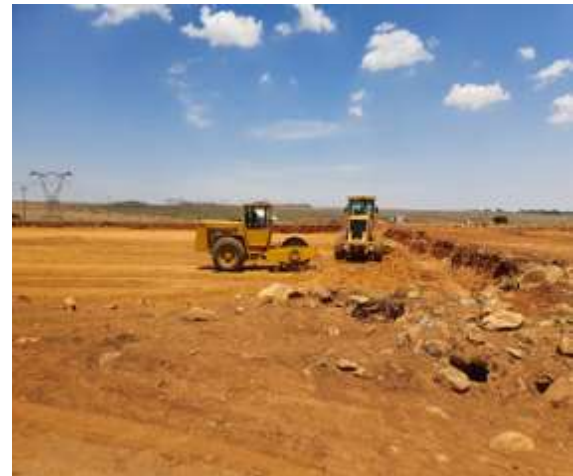
Figure 12: Backfilling and layering works for switching station footprint ongoing.
