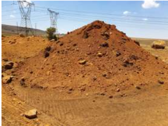
Figure 13: Topsoil stockpile stored onsite for rehabilitation purposes.
