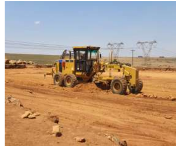
Figure 11: Backfilling and layering works for switching station footprint ongoing.
