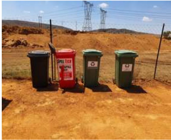
Figure 7: Spill kit and waste bins for waste segregation available at site camp.
