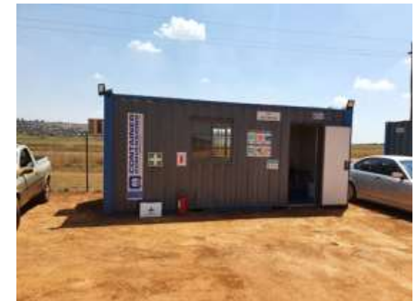
Figure 6: Office container with first aid kit and fire extinguisher available at site camp.
