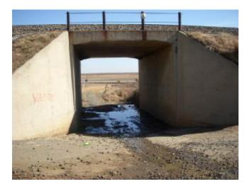
Figure 2. Water logging concern with normal culverts.
