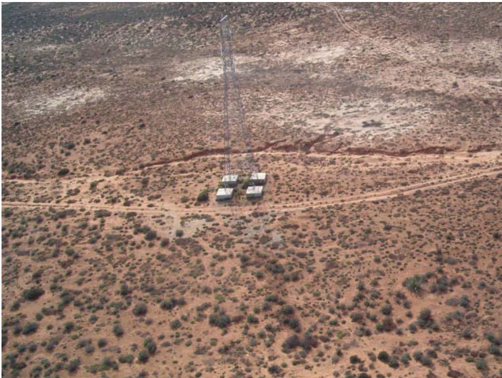
Figure 4: Pronounced water erosion along the existing ESKOM servitude as a result of preferential water flow in an old service road.
