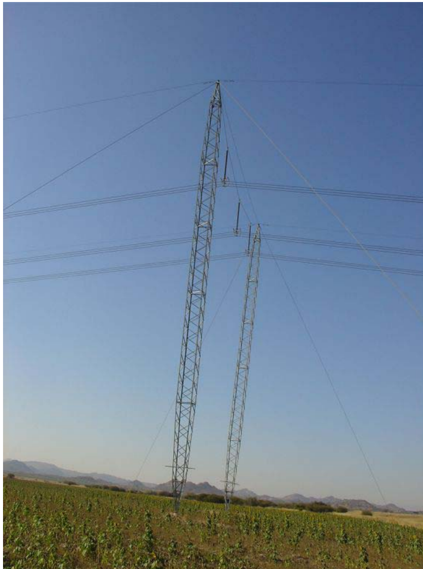
Figure 6: Example of a crossrope suspension pylon with a very small footprint near Pilansberg in the Northwest.
