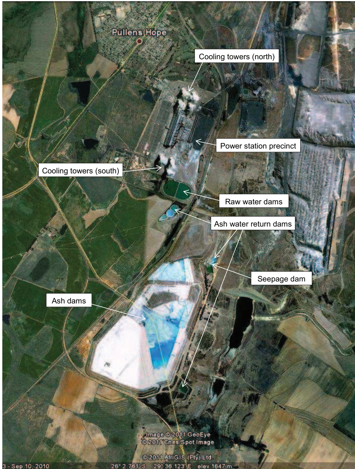
Figure 1: Location of Hendrina Power Station, Mpumalanga showing various infrastructure (courtesy Google Earth)
