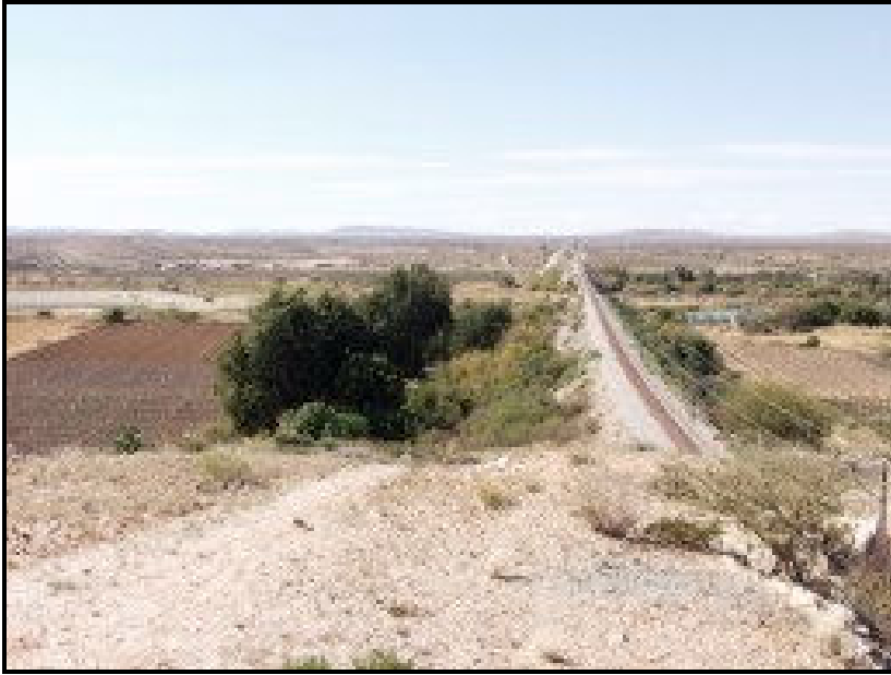
Orange River crossing near railway line – looking north
