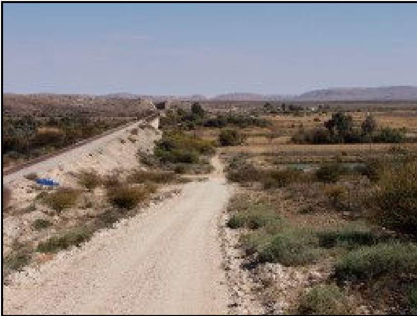
Orange River crossing at railway line – looking south
