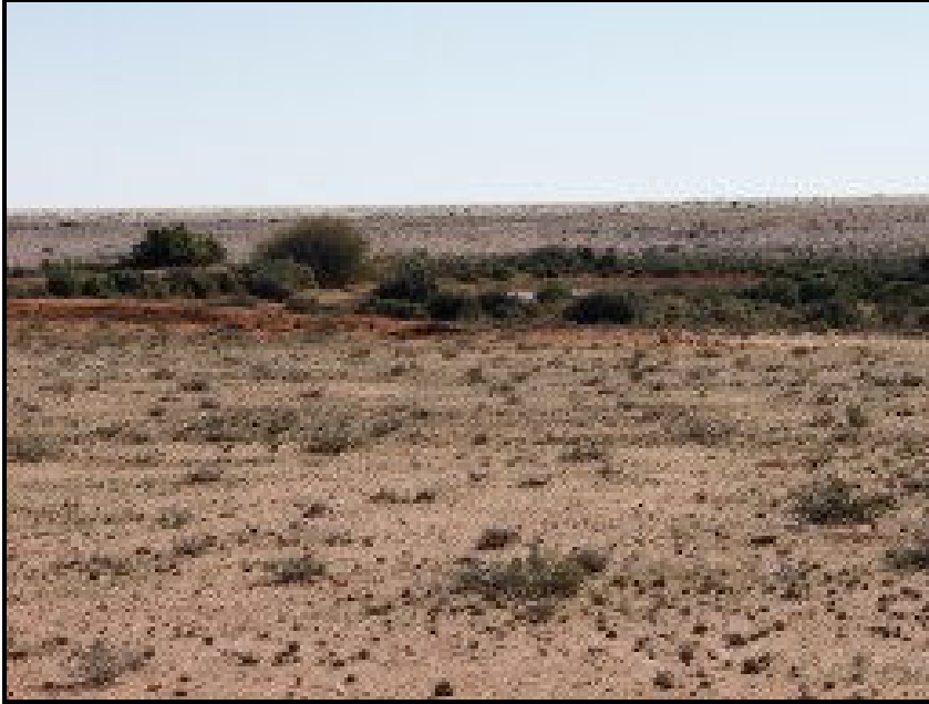
Typical small earthen dam along the alignment
