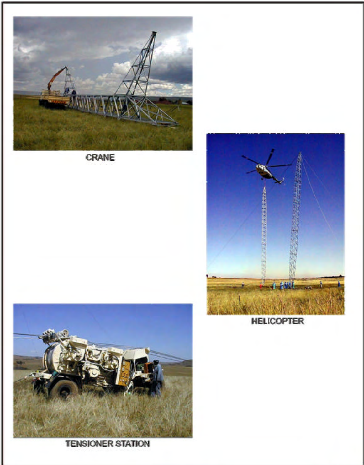
Figure 3: Typical construction equipment
