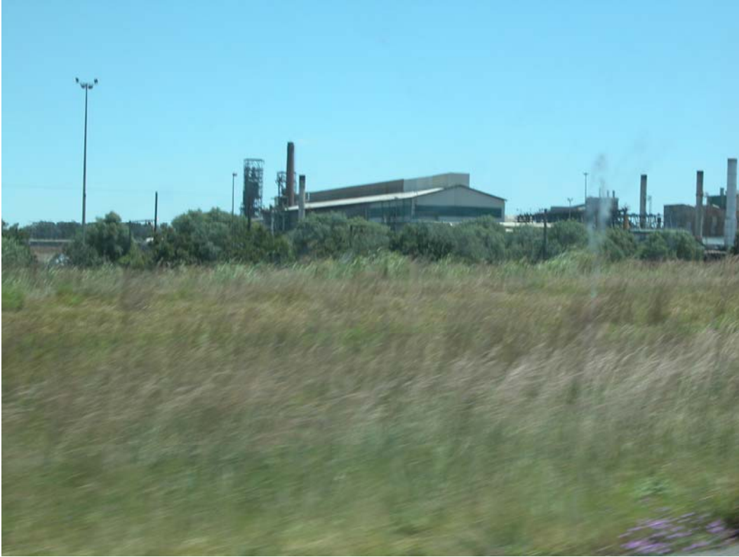
FIGURE 5: Industrial area near Glockner substation
