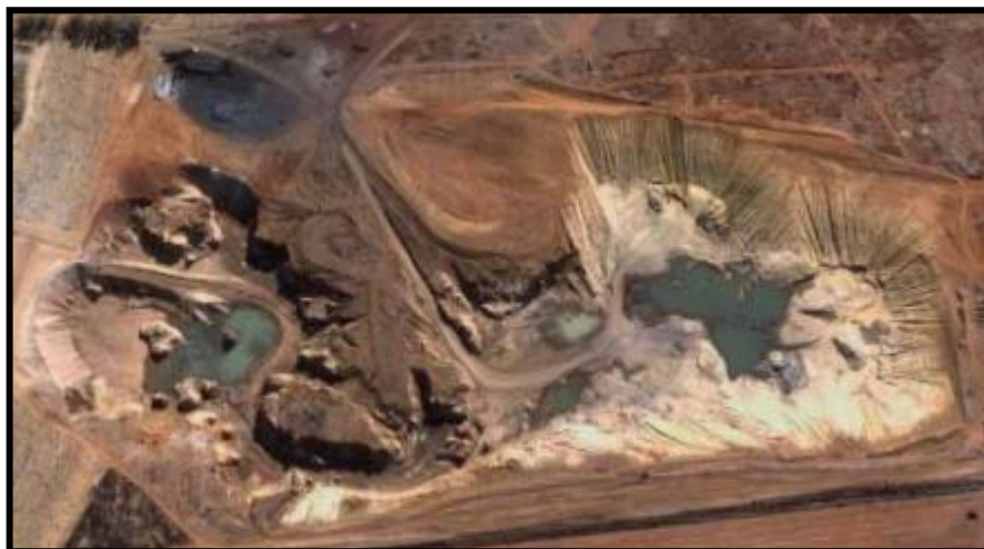
FIGURE 6: Dams associated with quarries
