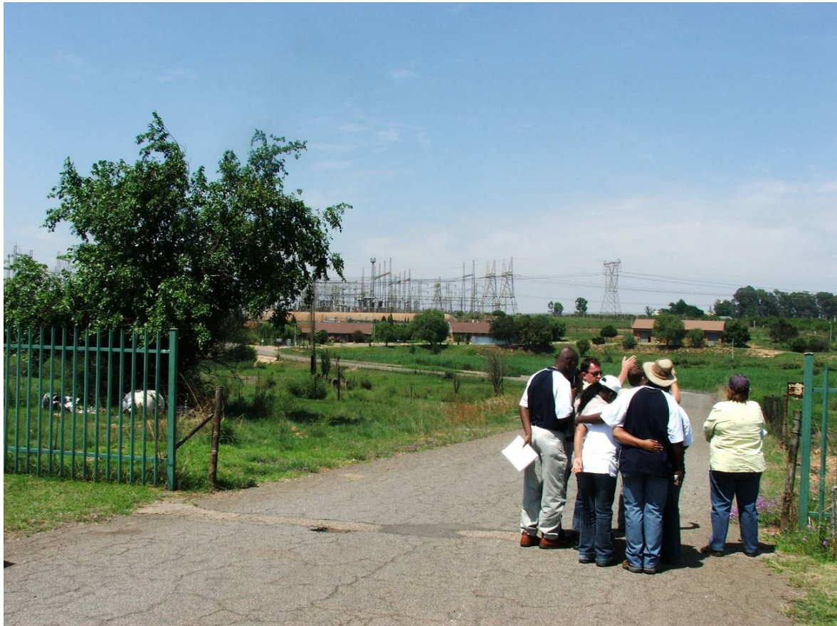
Photo 1. Glockner sub station
