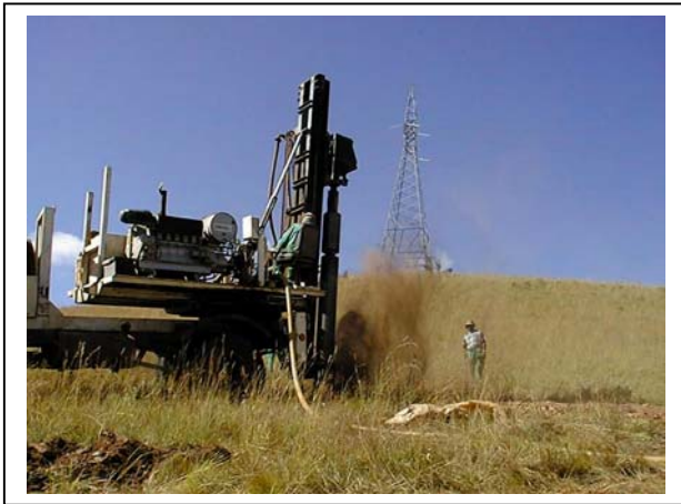
Photograph B3: Drilling of foundations
