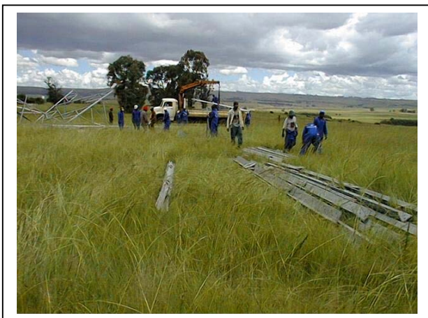
Photograph B5: Towers are erected on site
