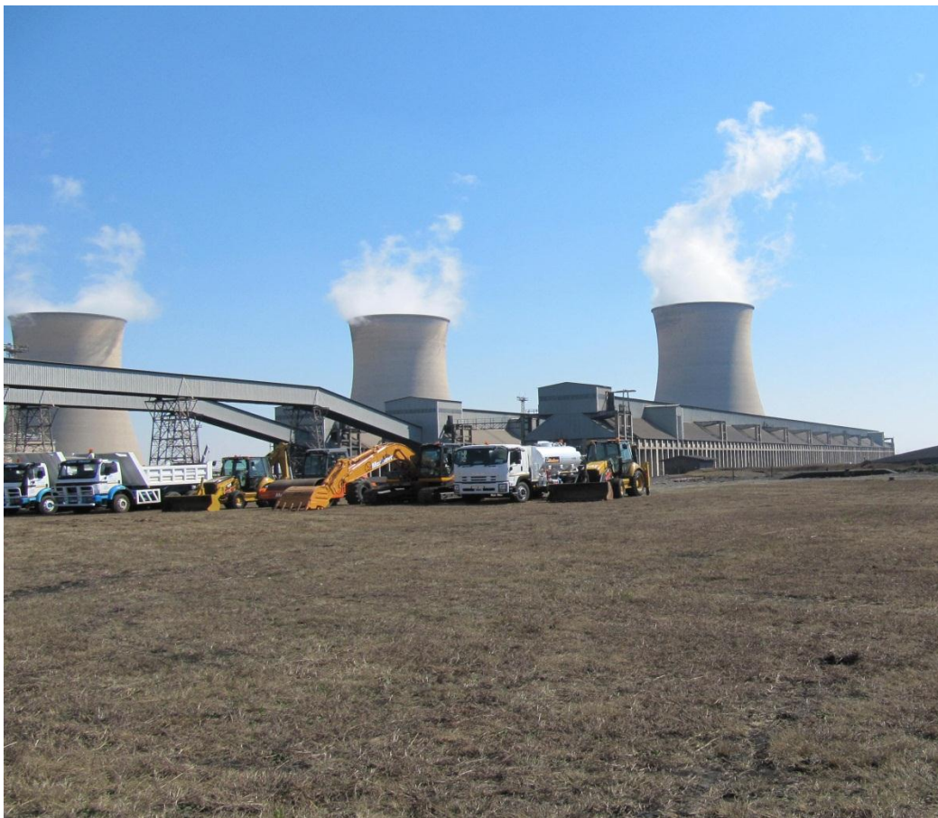
View looking north west
