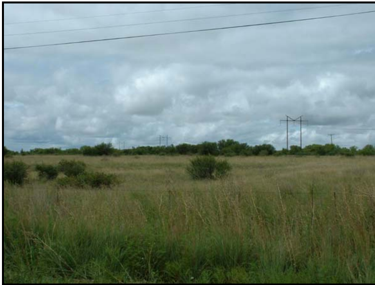
Figure 12. Existing overhead powerline at crossing point of Alternative 1 on the Vals River.
