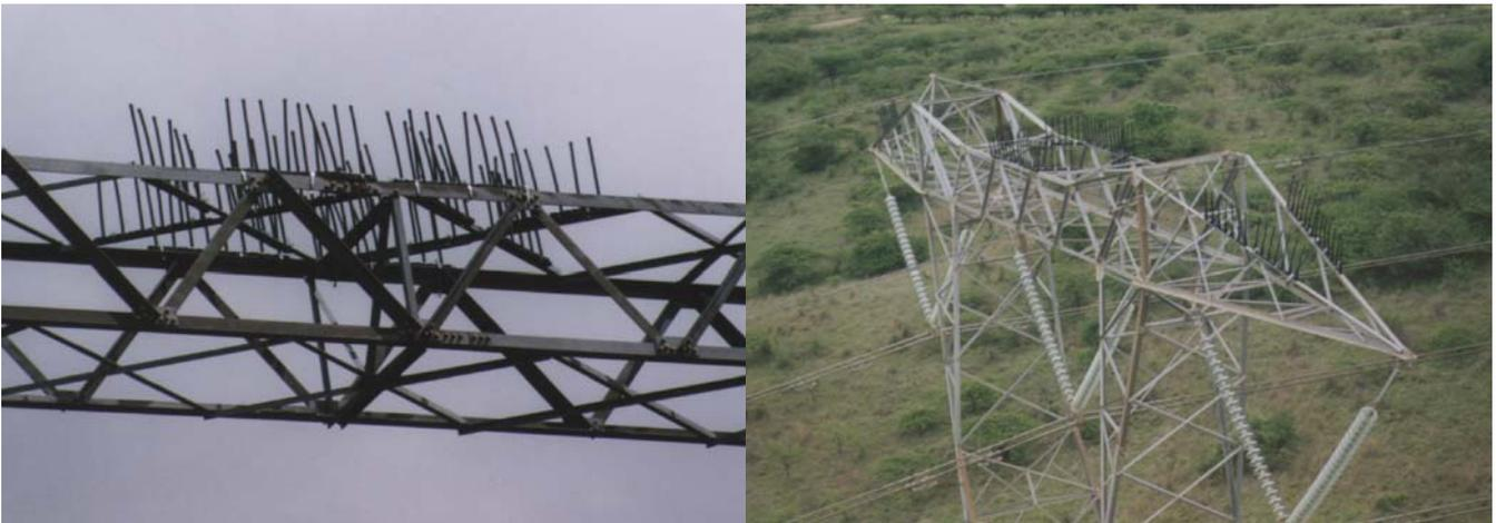
Figure 17: Photos showing the fitting of “Bird Guards” to the self-supporting tower structures.
