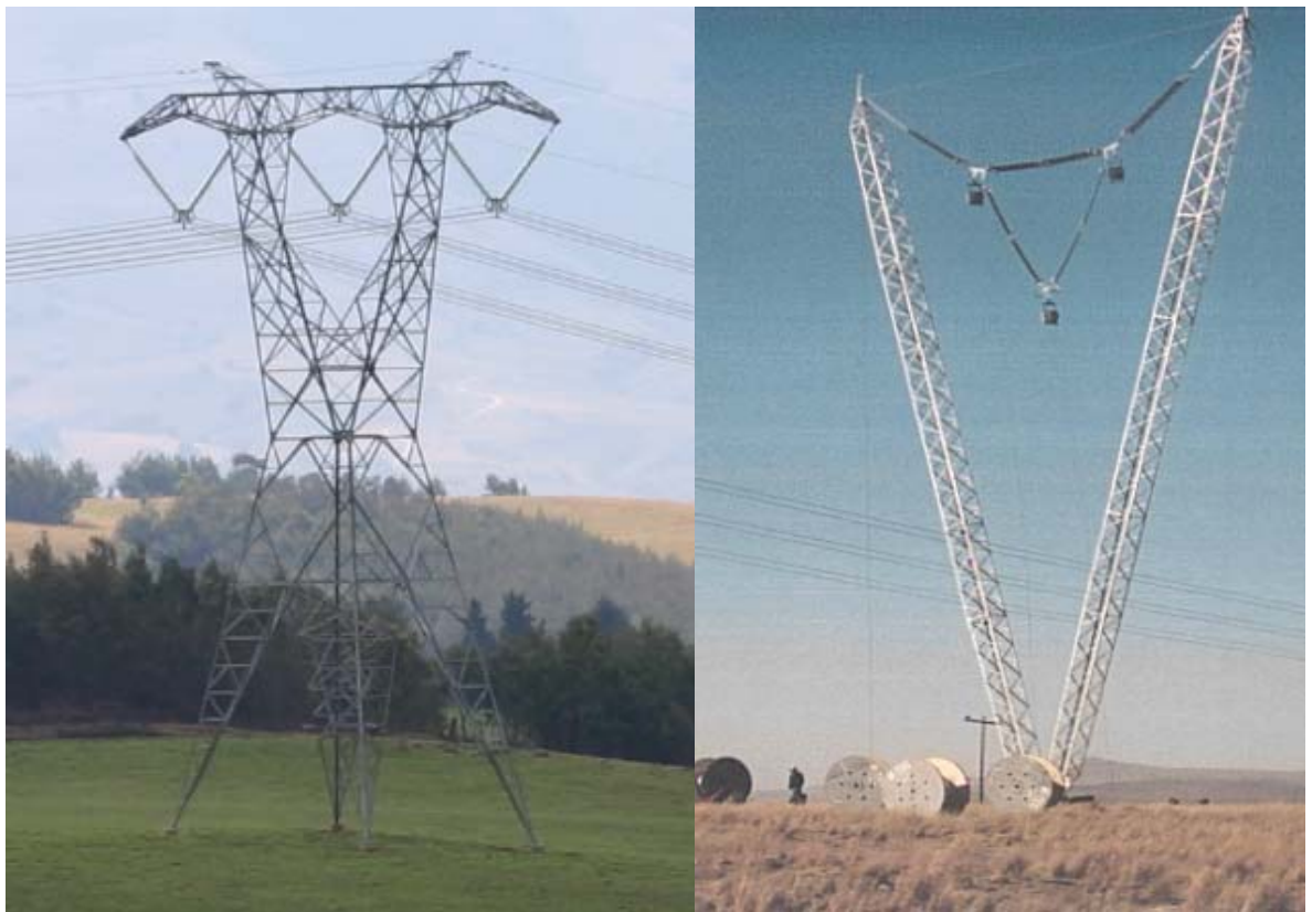
Figure 2c: Examples of both strain tower and compact cross rope suspension tower types
