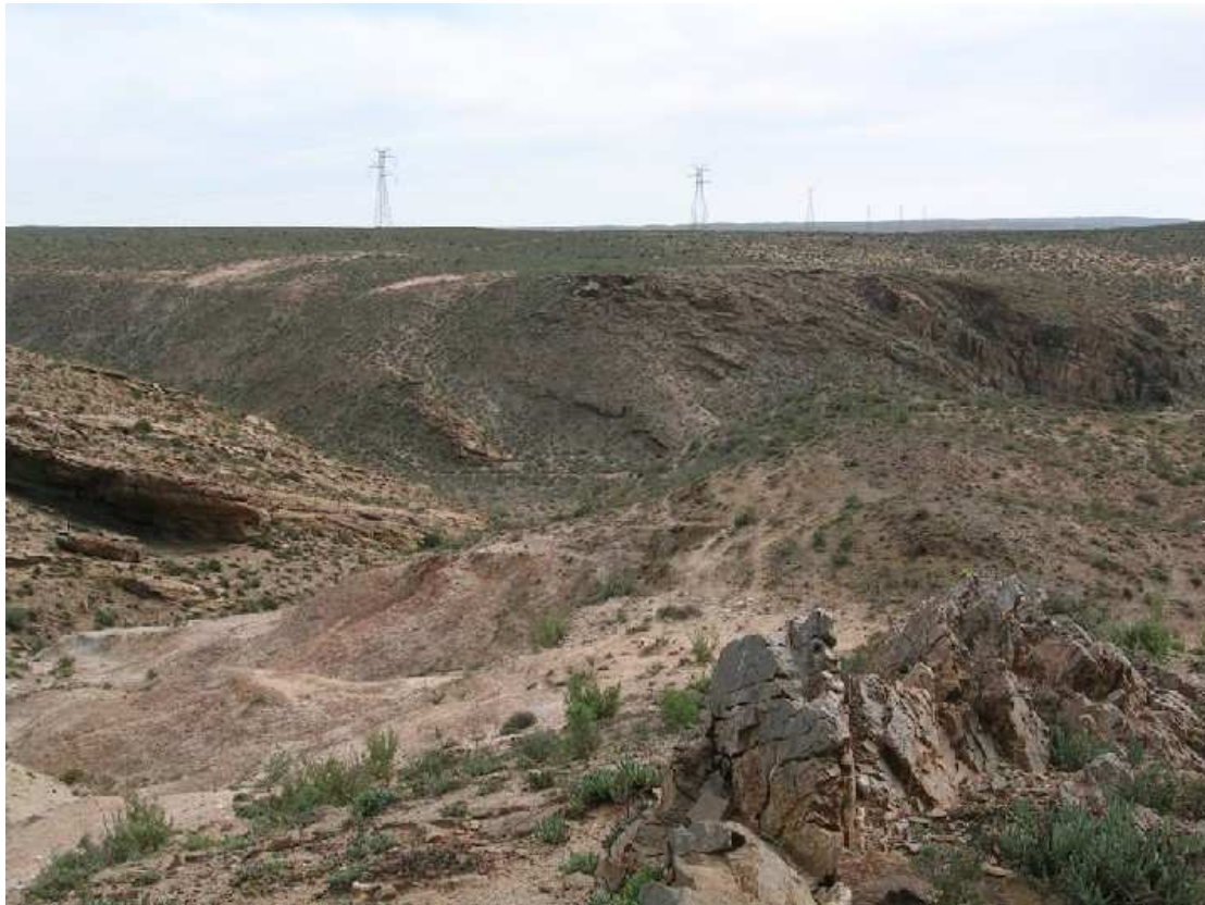
Plate 3: View north across Holgat River gorge, showing existing powerline and High sensitivity rocky outcrops. The service track runs to the right of the photo.
