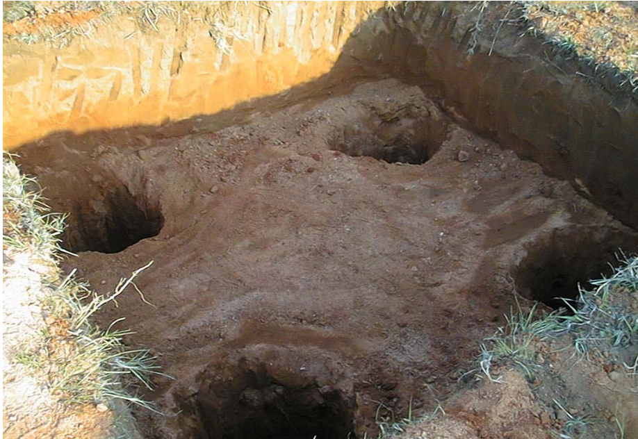
Figure 3.4: Example of a tower foundation
