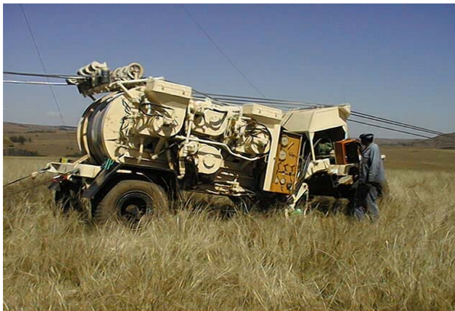
Figure 3.5: Mechanical stringing of the conductors
