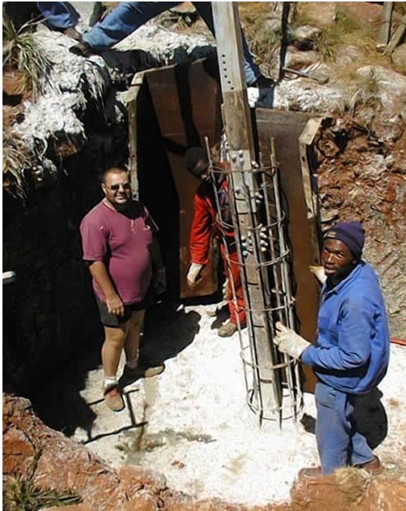
Figure 3.3: Tower foundation construction
