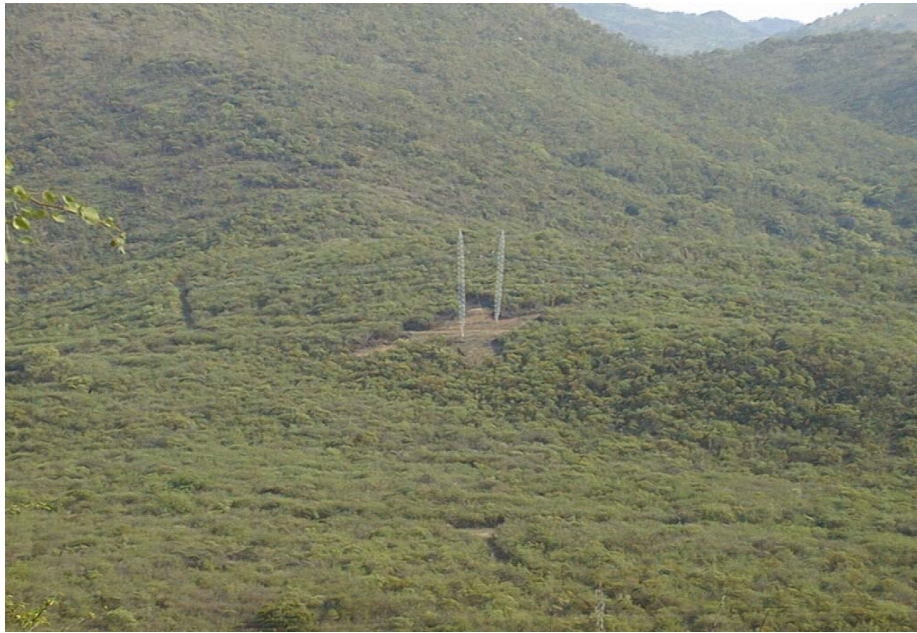
Figure 3.1: Example of Bushclearing around a Transmission line tower
