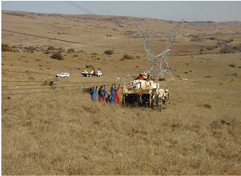
Figure 3.6: Mechanical stringing of the conductors
