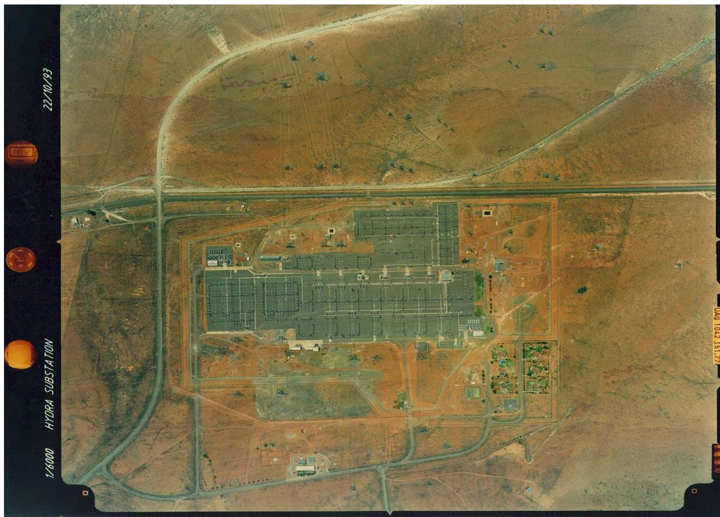
Figure 4.4: Existing Hydra Substation with existing access road on western side of substation.
