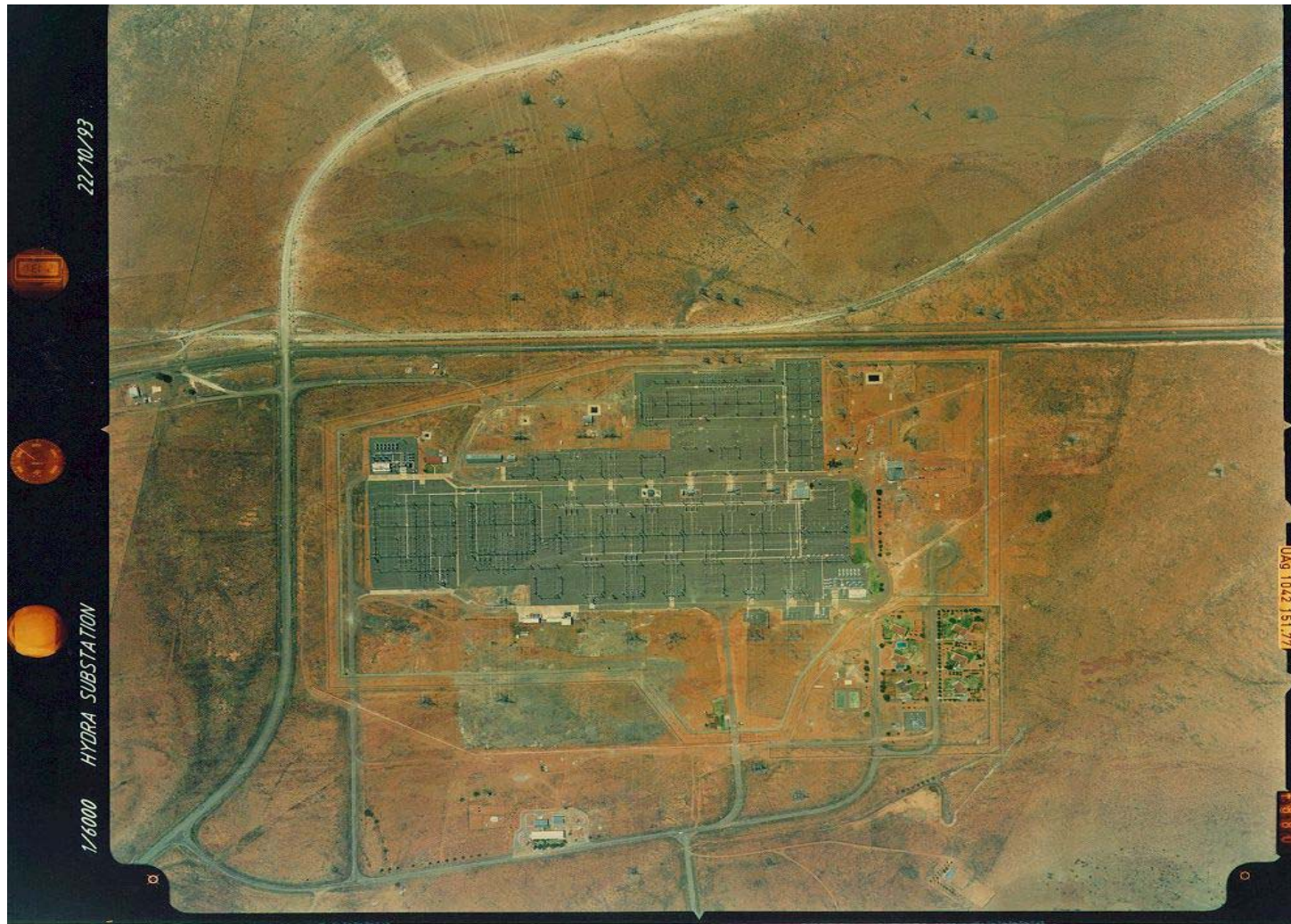
Figure 4.3: Existing Hydra Substation with existing access road on western side of substation.
