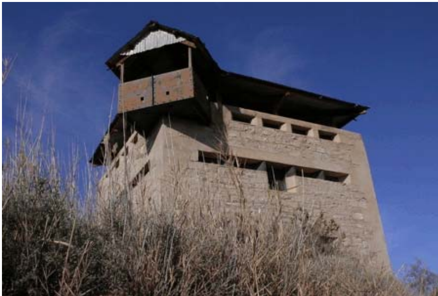
Photograph 6.5: Masonry blockhouse at Merriman close to Deelfontein
