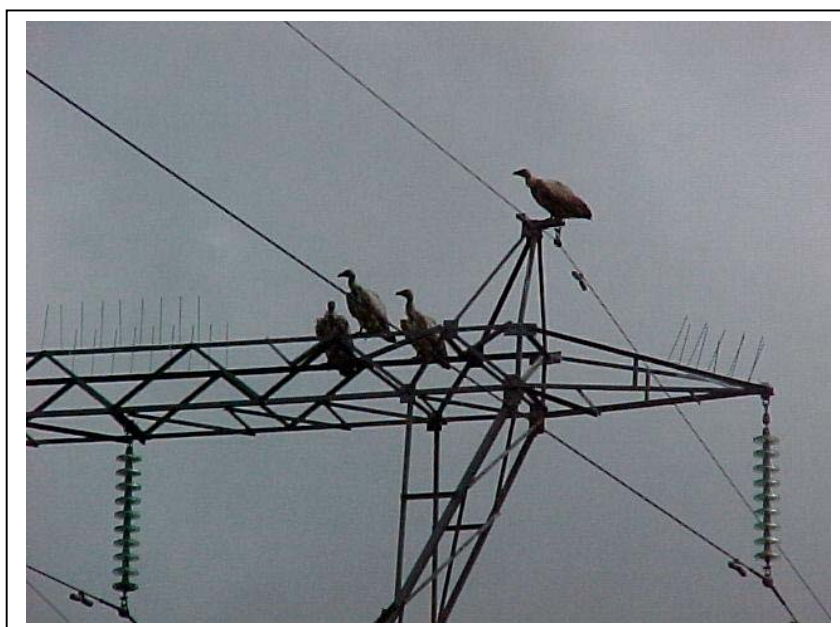
Figure 4.4: Bird guards should be implemented in areas where the streamer effect could pose a threat to the reliable operation of the powerline
