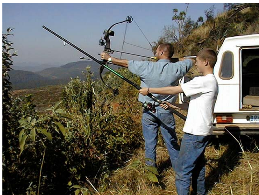
Photograph 2.4: Alternate stringing methods, such as the use of a bow and arrow, will be implemented in sensitive areas
