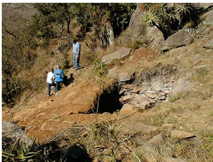
Photograph 2.5: Where areas are inaccessible, foundations will be dug by hand
