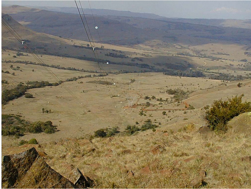
Photograph 9.1: Bird diverters have been developed and have effectively reduced the incidents of bird collisions with Transmission lines
