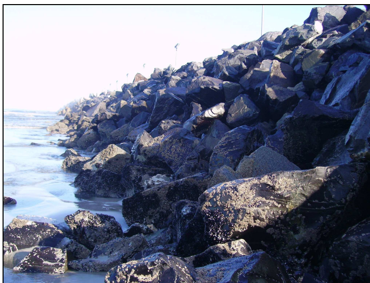
Figure 2. The exposed seaward side of the Koeberg breakwater
