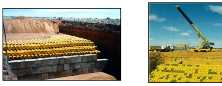
Figure 3-5: Disposal of Low Level Radioactive Waste steel drums at Vaalputs. The drums are covered with layers of clay
