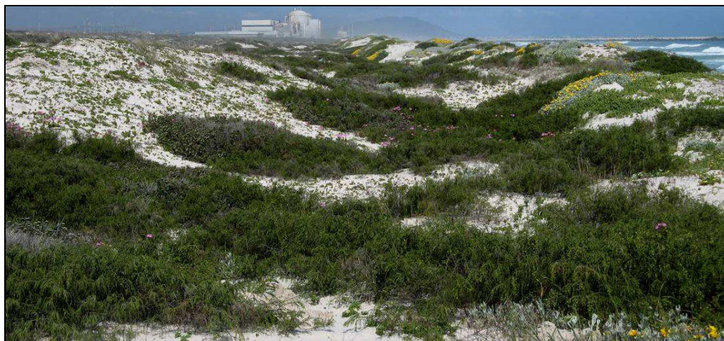
Figure 8-23: A view of the affected environment at the Duynefontein site, looking south towards Koeberg Nuclear Power Station
