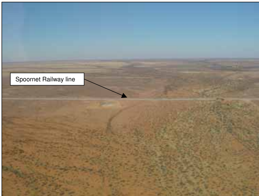
Figure 7. An aerial view of the railway line located within the study area.
