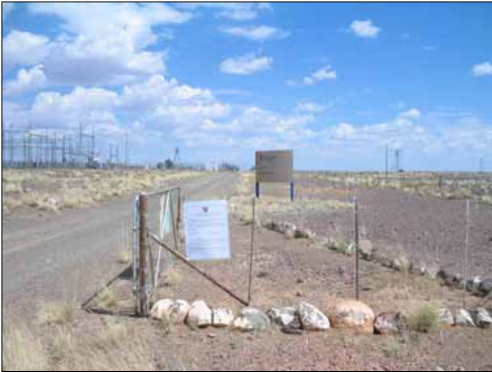
Aries substation site notice
