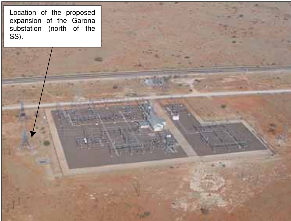
Figure 3. An aerial view of the Garona Substation located in the northern section of the study area (showing the location of the proposed extension).
