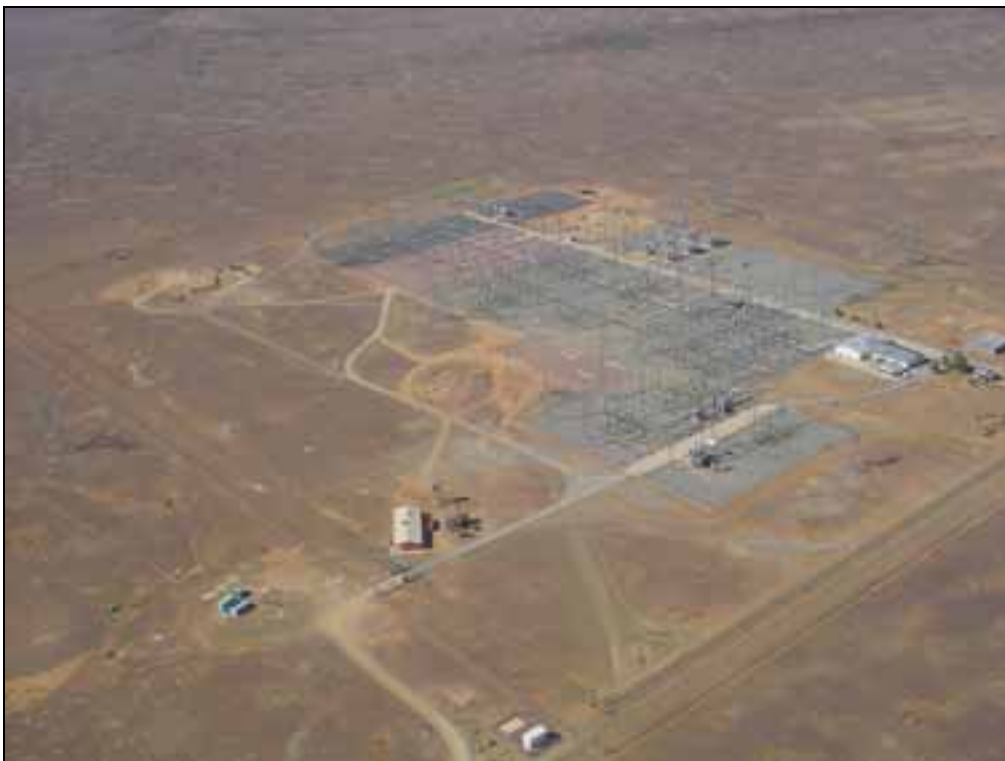
Figure 4. An aerial view of the Aries Substation located in the southern section of the study area.
