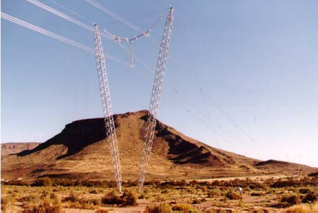
Figure 1: Photography of installed Compact Cross-Rope tower
