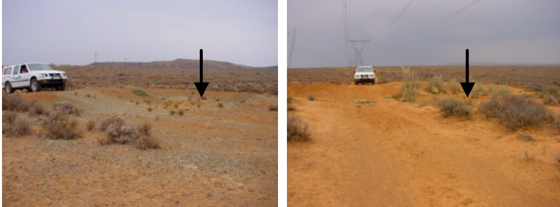
Figure 4. Examples of well constructed berms under the Hydra-Droërvier 1&3 lines. This design uses an overflow dam to spread water collected by the berm (see arrows). After ten years virtually no maintenance is required on these structures.
