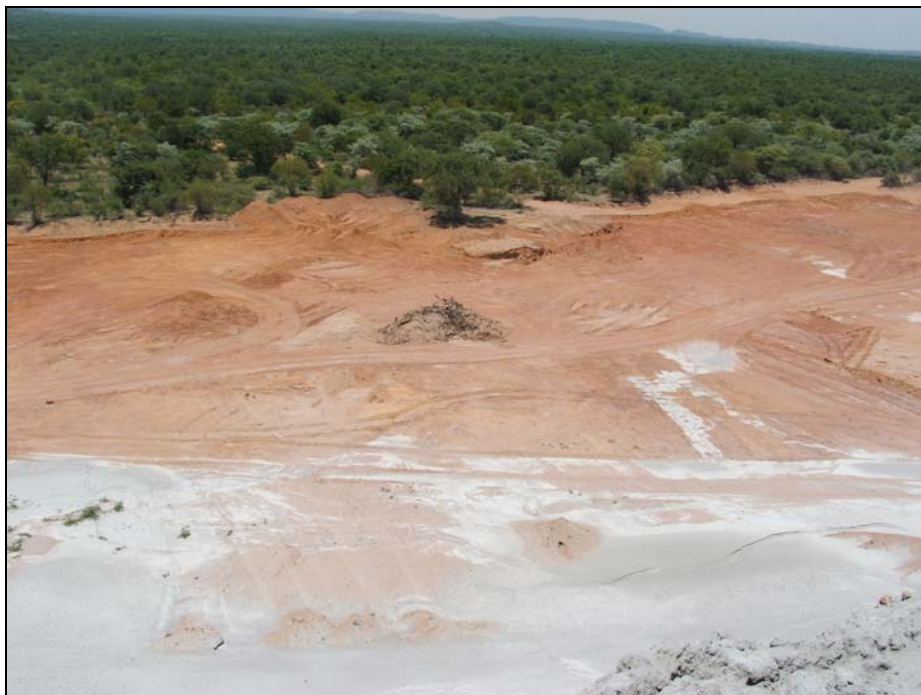
Figure 9.12: Borrow area located to the south of the existing ash dump at Zwartwater from where soil is removed for placement on the surface of the ash dump. The ash dump will expand into this area.
