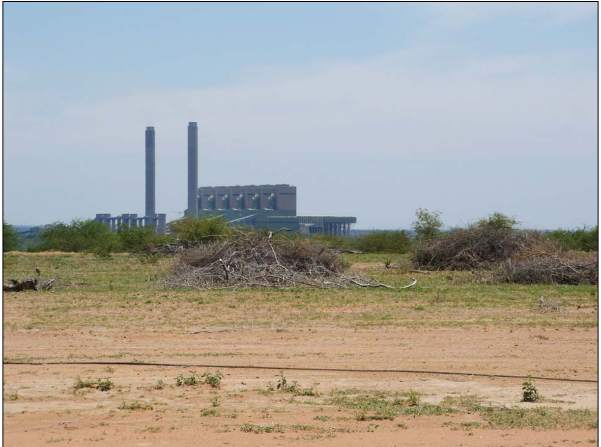
Figure 9.9: Existing Matimba Power Station showing the two 250 m stacks. Due to the particulate abatement measures implemented no visible plumes occur during routine operations.
