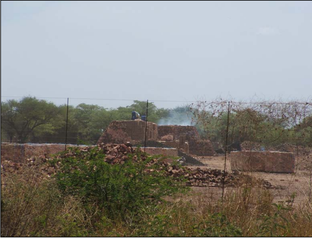
Figure 9.15: Firing by clamp at the brickmaking operations at Hanglip.
