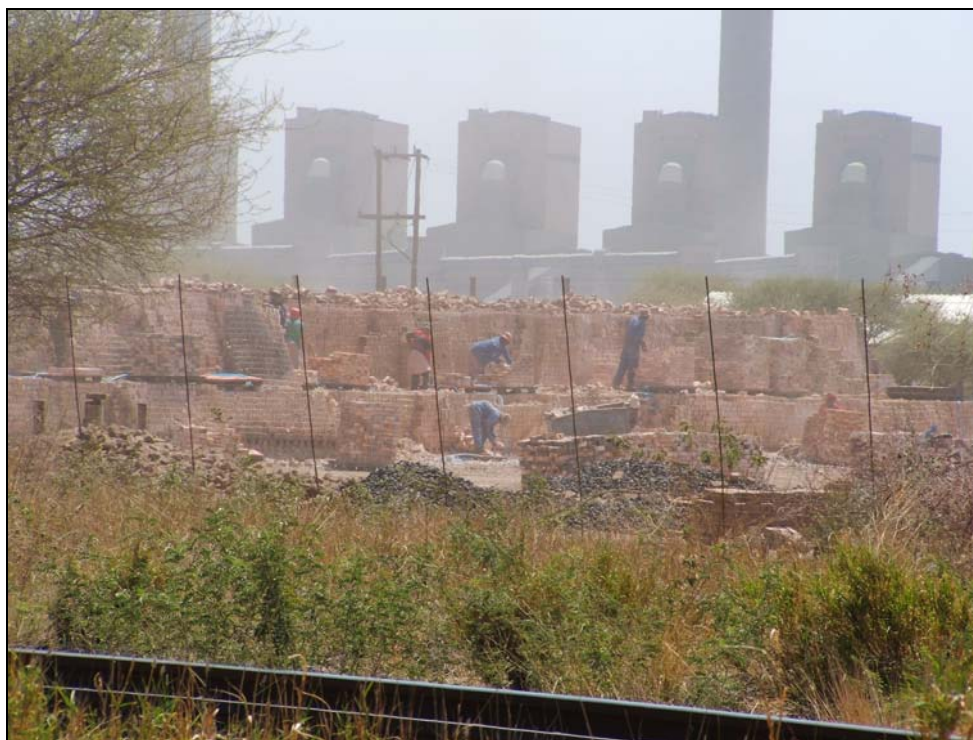
Figure 9.14: Operations at the brickworks at Hanglip located in close proximity to the Matimba Power Station (evident in background).
