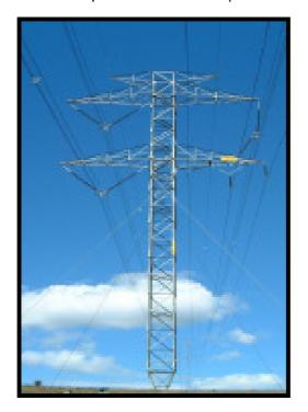
Photo 2: Self - supporting double circuit suspension tower.
