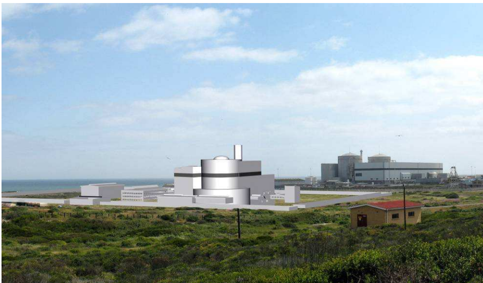
Photo 10: Visual mitigation – Dark band and light stack reduces visual scale of structures – Pebble Bed Nuclear Reactor as example
